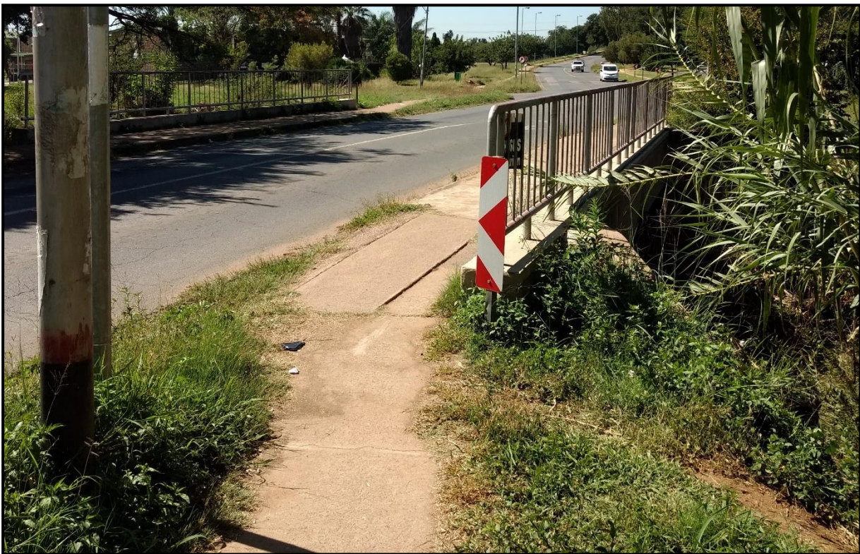
Figure C-2: Photograph of the Bridge where Vibration was Measured
