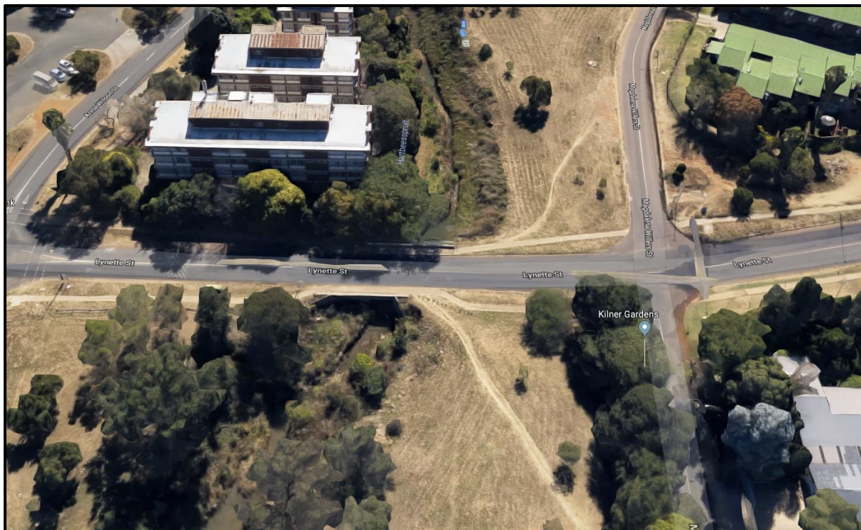
Figure C-3: Satellite Image of the Bridge on where Vibration was Measured
